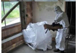
Asbestos/Lead Based Paint Removal Whittier, AK Client: US Forest Service
