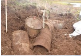
Drum Mound CON/HTRW Removal Action Umiat, AK Client USACE
