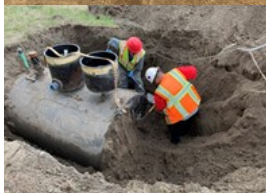
Tank Decommissioning and Closures Various Locations, AK Client: FAA
