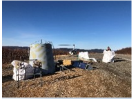
Remote Communications Outlet Decommissioning Mt. Fairplay, AK Client: FAA
