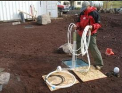
Installing a skimmer assembly for oil recovery from groundwater
