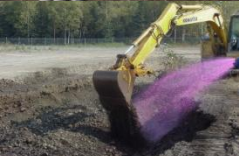
In-Situ Chemical Oxidation of Chlorinated Hydrocarbons (RCRA)
