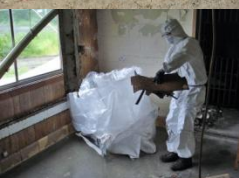
Asbestos/Lead Based Paint Removal
