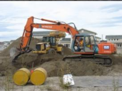
Excavating Munitions and Explosives of Concern (MECs)
