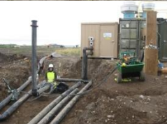
Installing a High Volume Vapor Extraction System
