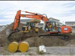
Excavating Munitions and Explosives of Concern (MECs)
