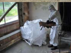
Asbestos/Lead Based Paint Removal
