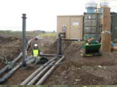
Installing a High Volume Vapor Extraction System
