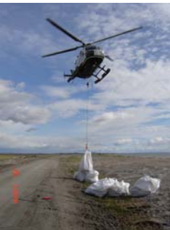
Helicopter being used to transport Geobags of contaminated waste.
