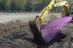
In-Situ Chemical Oxidation of Chlorinated Hydrocarbons (RCRA)
